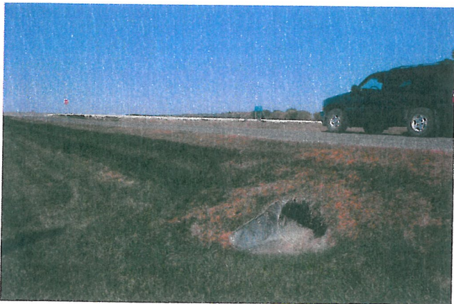
South side of CMP at Outfall 1, near Highway 76 – view facing north
