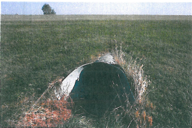
Outfall 2: Facing West – East edge of the Airport property (BML02).
