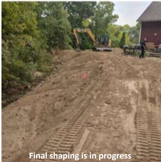
Clay fill being compacted on top of the geo textile blanket
