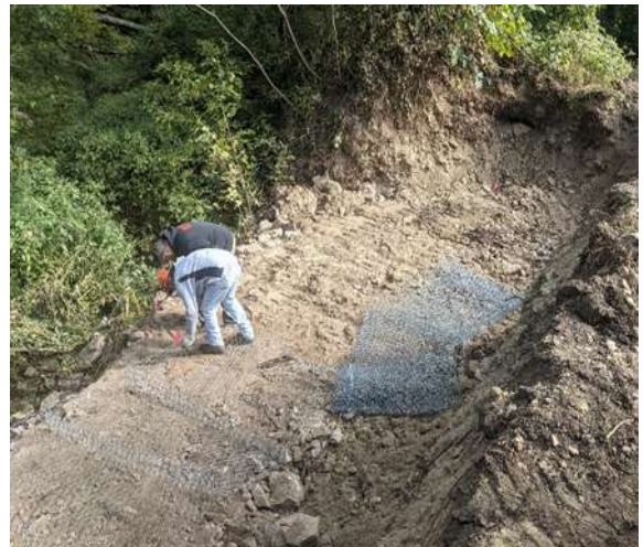
Gabion baskets being placed
