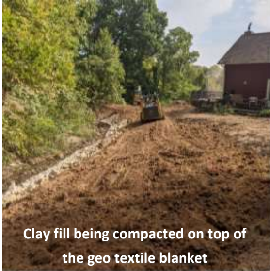
Earth fill is compacted over the clay fill
