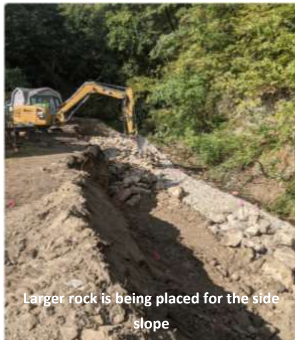
Larger rock is placed to anchor the smaller rock
