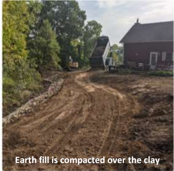
Clay fill being compacted on top of the geo textile blanket
