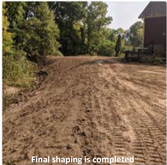
Earth fill is compacted over the clay fill
